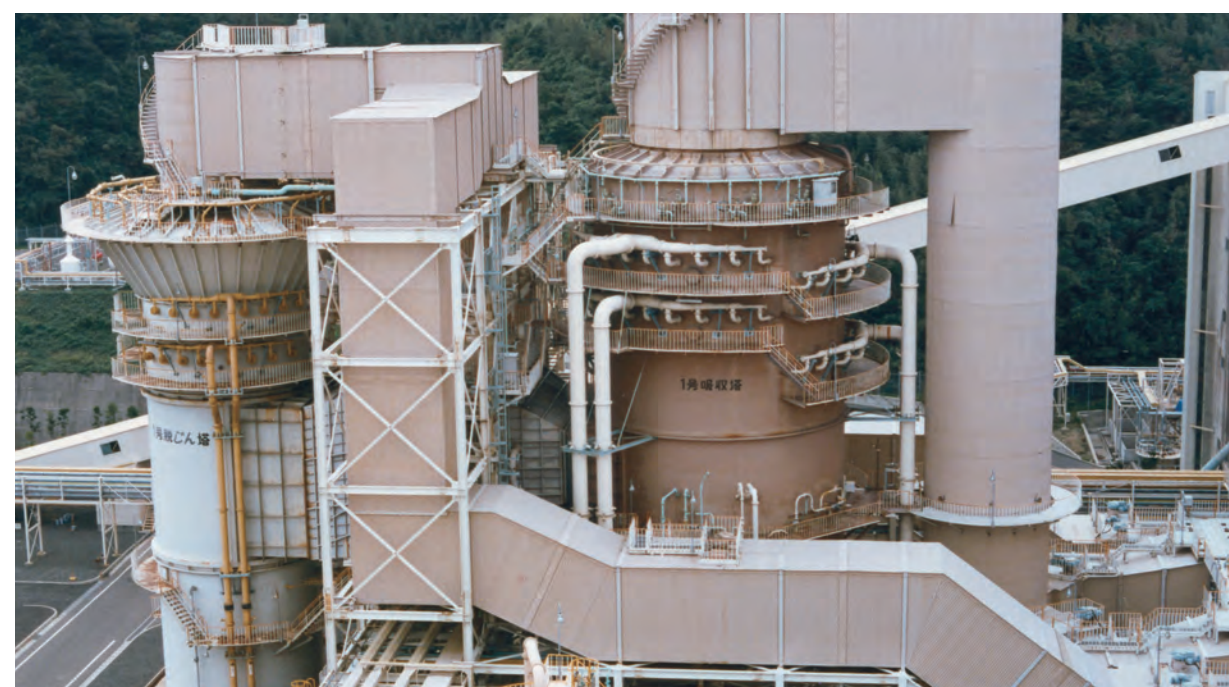
Flue gas desulfurizer absorption column and cooler — FUJI FLAKE AC
